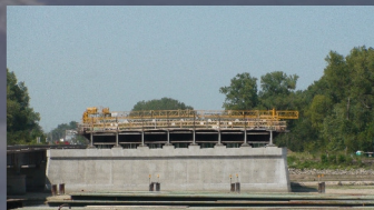
Fremont, NE 427m x 24m Prestressed Beam Bridge
