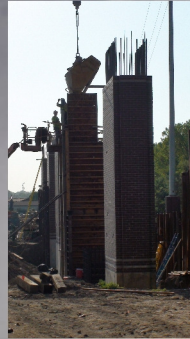
Sioux City, IA Brick Faced Pier Columns Kelly, Darren, Scott C, Scott D. and Bob are making a big push to get traffic on 2 bridges over I-29.
