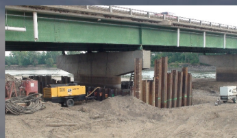
Ottumwa, IA 770' x 77' Steel Girder Bridge
